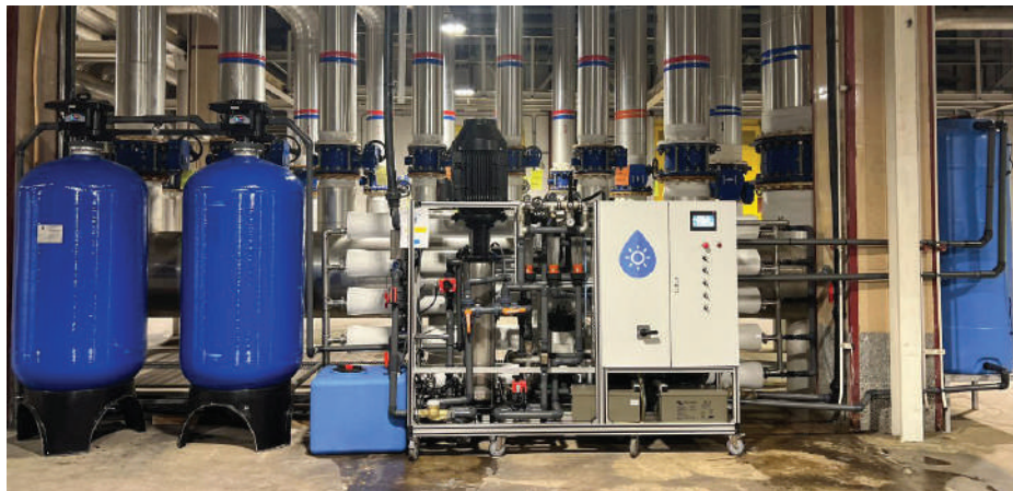
Solar Water Desalination System, South Iraq, 50cmh, 120 kWp Solar Panels
